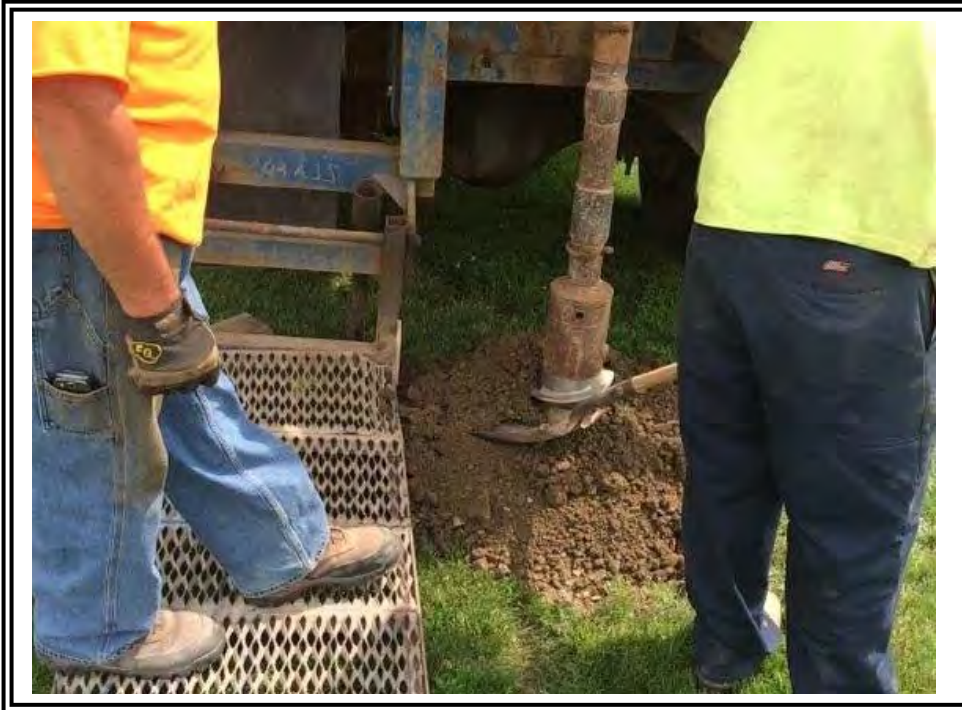
Drilling Operations at Boring B-2
