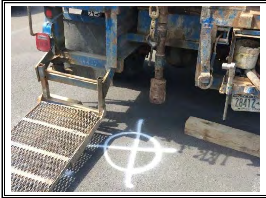
Drill Rig Mobilized at Boring B-4
