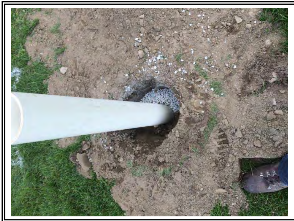
PVC Pipe Installation for Infiltration Testing at Boring B-3
