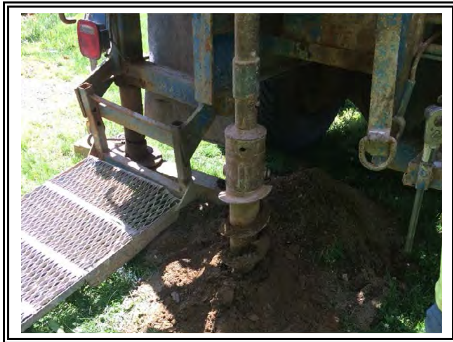
Drilling Operations at Boring B-5
