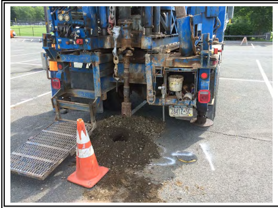
Drilling Operations at Boring B-1
