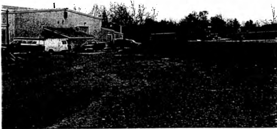
Photograph 3 (Roll 1, Neg. 9) View northeast from the Physical Plant, showing the cut and filled area of the track field.
